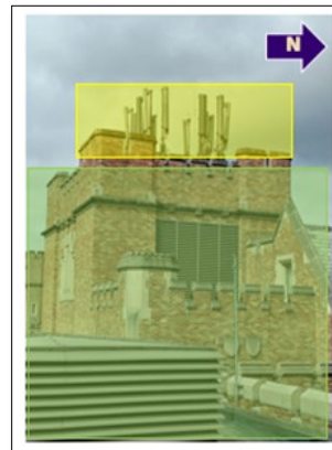
Figure 2: Main roof - Category 1
