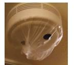
devices could be removed, bagged or otherwise disabled. Duct detectors and other devices that may be hidden can be identified through record drawings.
