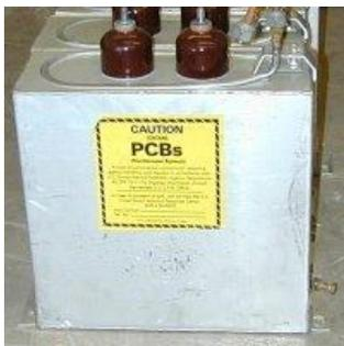
Remodels, laboratory moves, and standard maintenance and alterations work all require that equipment suspected or known to contain PCBs be inspected and screened for PCB contamination. Examples of items include old x-ray machines and other large older laboratory equipment that contain power sources, power generators and capacitors (pictured), as well as fluorescent light ballasts.
